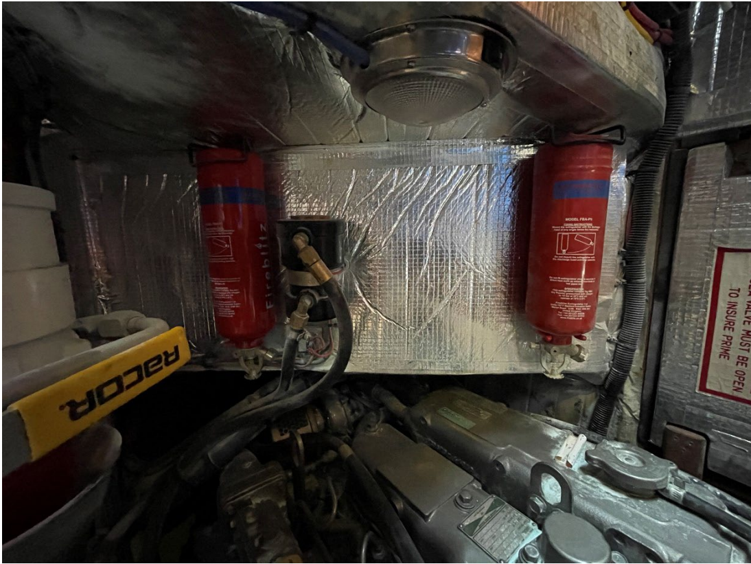
Fig. 1: Only the fire extinguisher on the right of the picture had fired. This photograph was taken after the initial cleaning with the dinghy pump.
