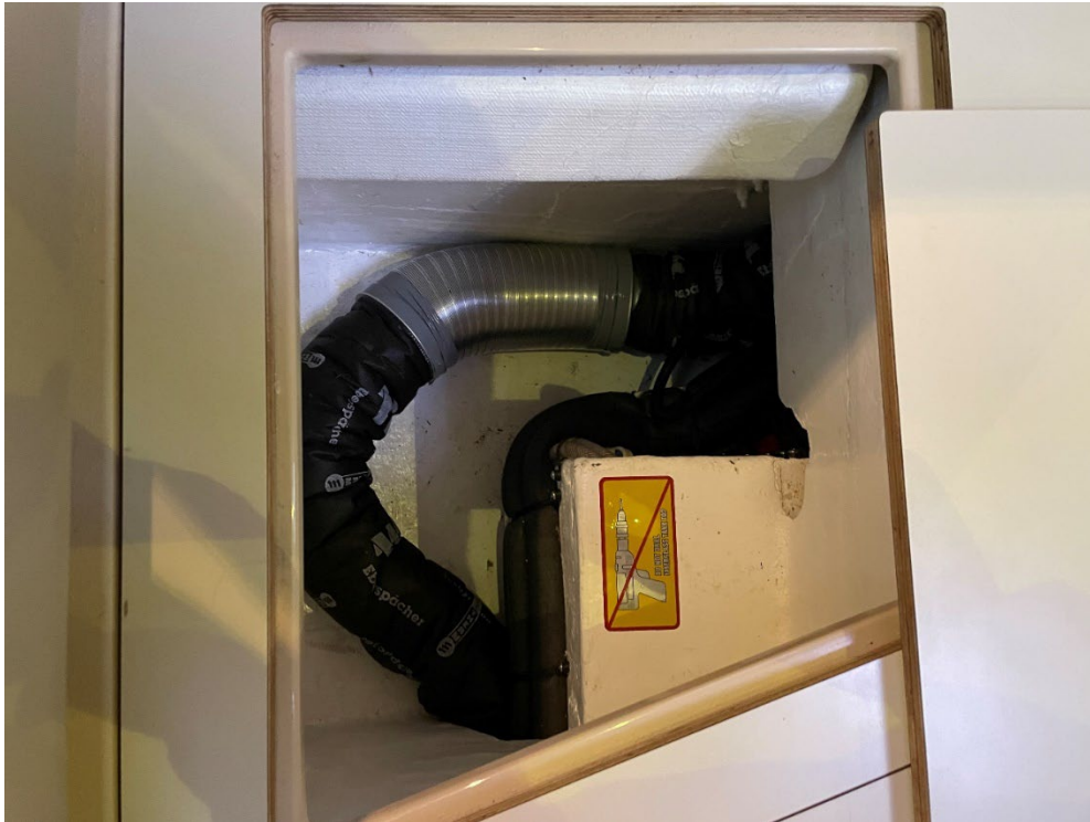
Fig. 11: The ducting installation in the locker below the starboard settee has been left lying on the floor. This position means it's impossible to use this space for storage now. It would have been much better to mount the ducting higher up on the outside locker walls, keeping the bottom clear, so this sizeable locker space could still be used without the duct getting damaged.
