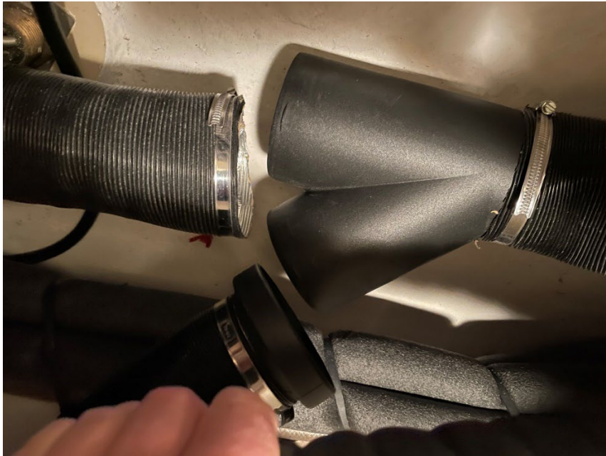
Fig. 8: Close-up of Y-connector. Both connectors had become detached as pictured. The hot air was being blown directly into the port side of the engine bay.
