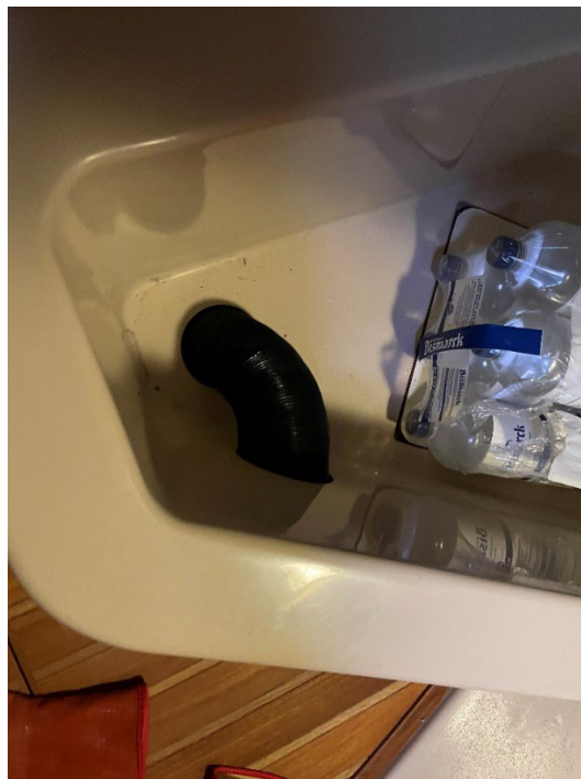
Fig. 10: The heater duct in the outboard quarter berth locker is badly exposed to being bashed around by whatever is stored there, emergency water in this instance.
