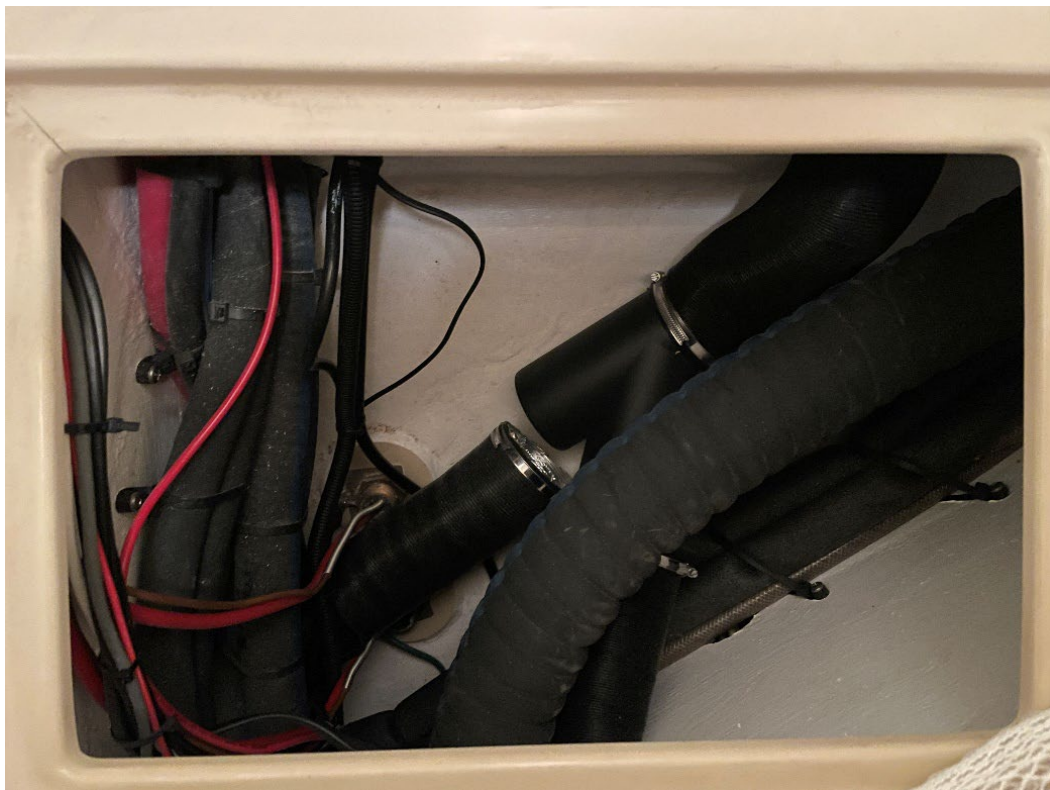
Fig. 7: The inboard quarter berth locker with the Y-connector in the heating duct. The walls of this locker were too hot to touch. The hole to the engine for pipework was to the bottom left of the picture.
