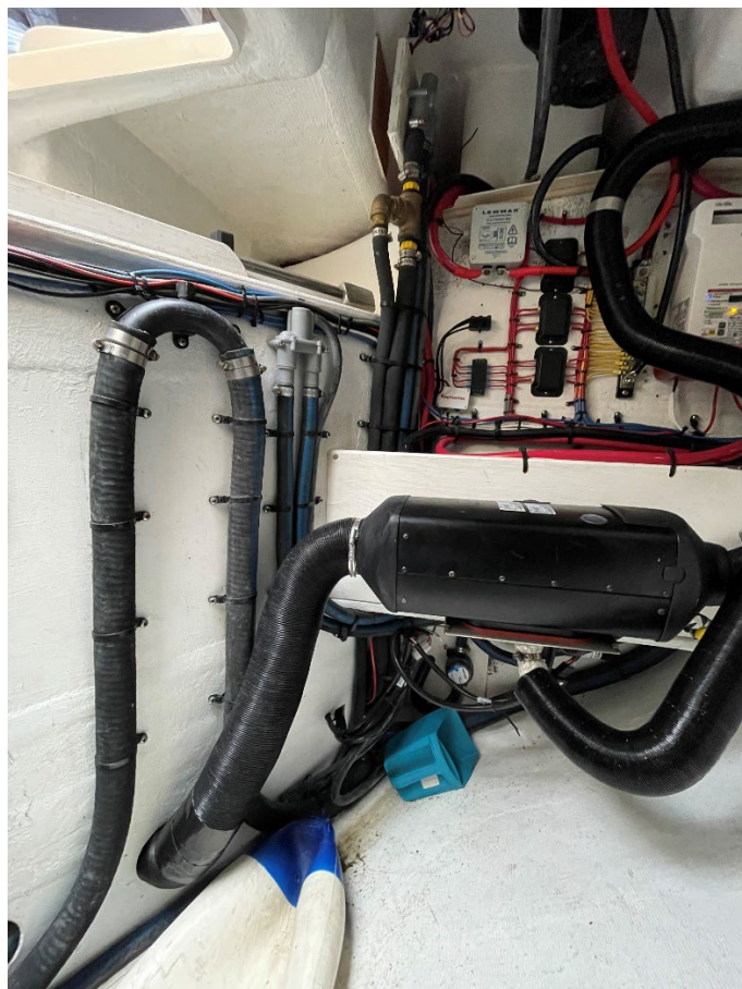
Fig. 9: The heater in the cockpit locker. Notice how securely fitted the bilge pump pipes are compared to the retro fitted heater duct. As well as being well secured to the bulkhead this section of ducting should have been of a stronger material, or had a guard made around it, to prevent if from being damaged by items stored in the locker. The tape at the bottom is our repair to a 3" tear in the duct.
